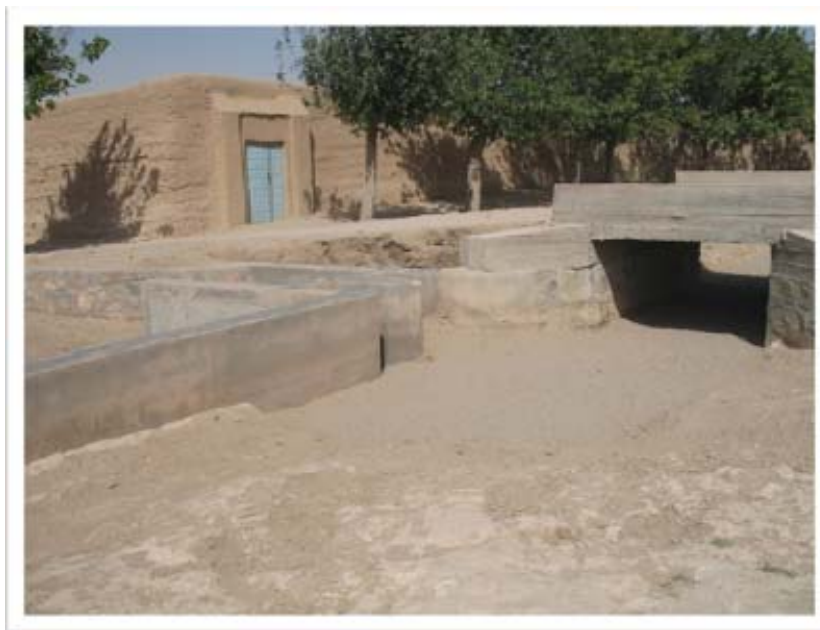
Illustration 3: Culvert Constructed with CDC funds, Pashtun Zarghun District, Herat
